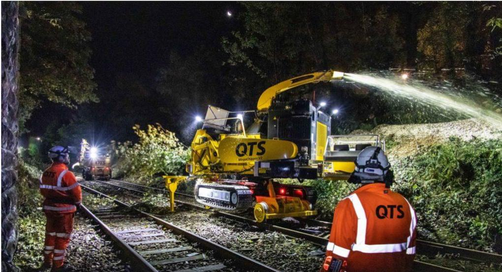
The Mega Chipper V2, part of QTS' 47-strong vegetation fleet, is currently being used on the East Kilbride line, which is undergoing electrification works. This six-month long project will see QTS work along 16 track miles, clearing all vegetation from both sides of the track by six metres, removing any dead, dying and dangerous trees which pose a risk to the infrastructure.
